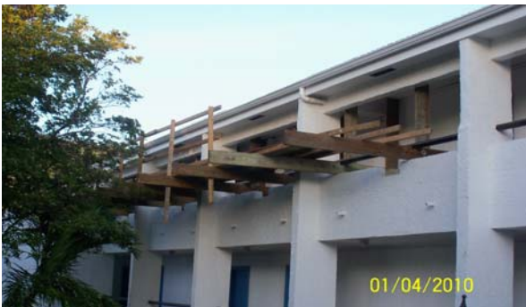
Scaffolding placed on Villas III top floor
