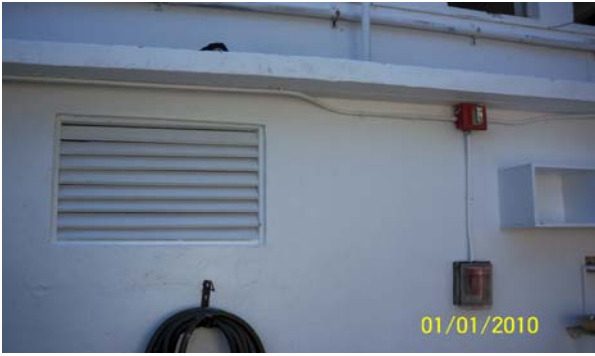
REPLACED WINDOWS IN MAINTENANCE BATHROOM
