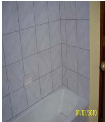
Bathroom tile complete on third and fourth floor
