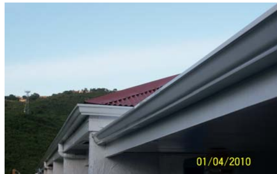
Gutter work beginning
