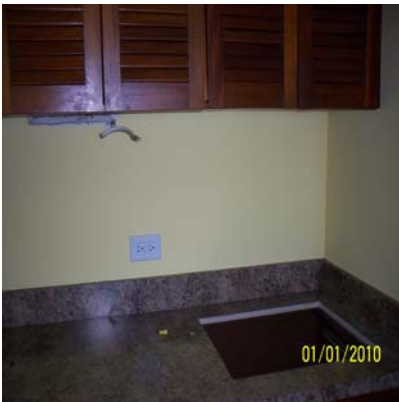
Counter tops back in place
