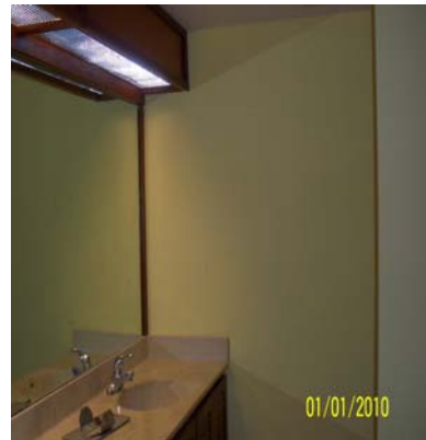
Sink tops set back in place
