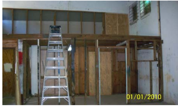
MAINTENANCE AREA PREPARED FOR HOUSEKEEPING RENOVATIONS
