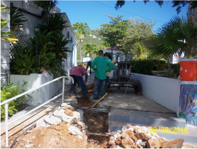
RUNNING NEW CONDUIT UNDER LOBBY COURTYARD FOR NEW PBX LINES
