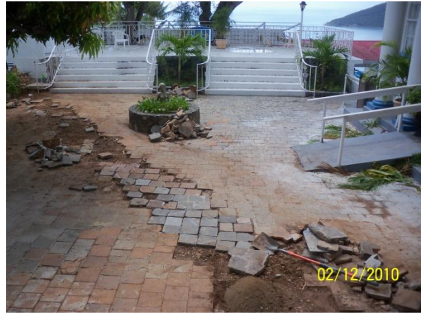
RUNNING NEW CONDUIT UNDER LOBBY COURTYARD FOR NEW PBX LINES
