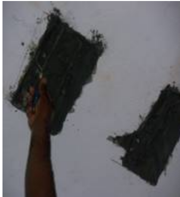
CONCRETE STRUCTURE REPAIRS IN FUTURE HOUSEKEEPING
