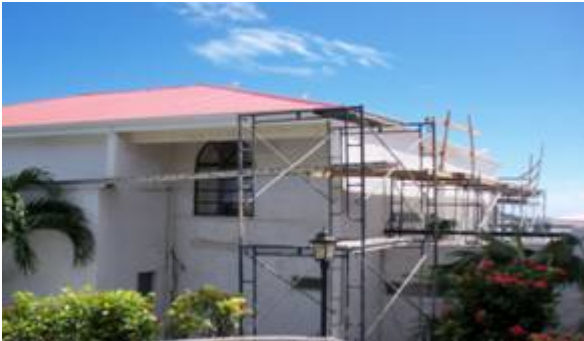
PREPARING TO CLOSE FOR REFURBISHMENT ON FEB 6TH.
