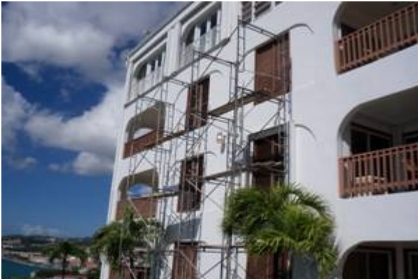
PREPARING SCAFFOLDING TO CHANGE OUT WUO WINDOWS AT END OF HILLTOP II TO INCLUDE UNIT 254
