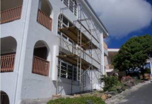
PREPARING SCAFFOLDING TO CHANGE OUT WUO WINDOWS AT END OF HILLTOP II TO INCLUDE UNIT 254
